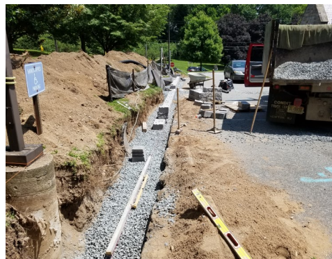
A new retaining wall and bluestone steps have replaced the old railroad tie construction, and new railings have been installed.
